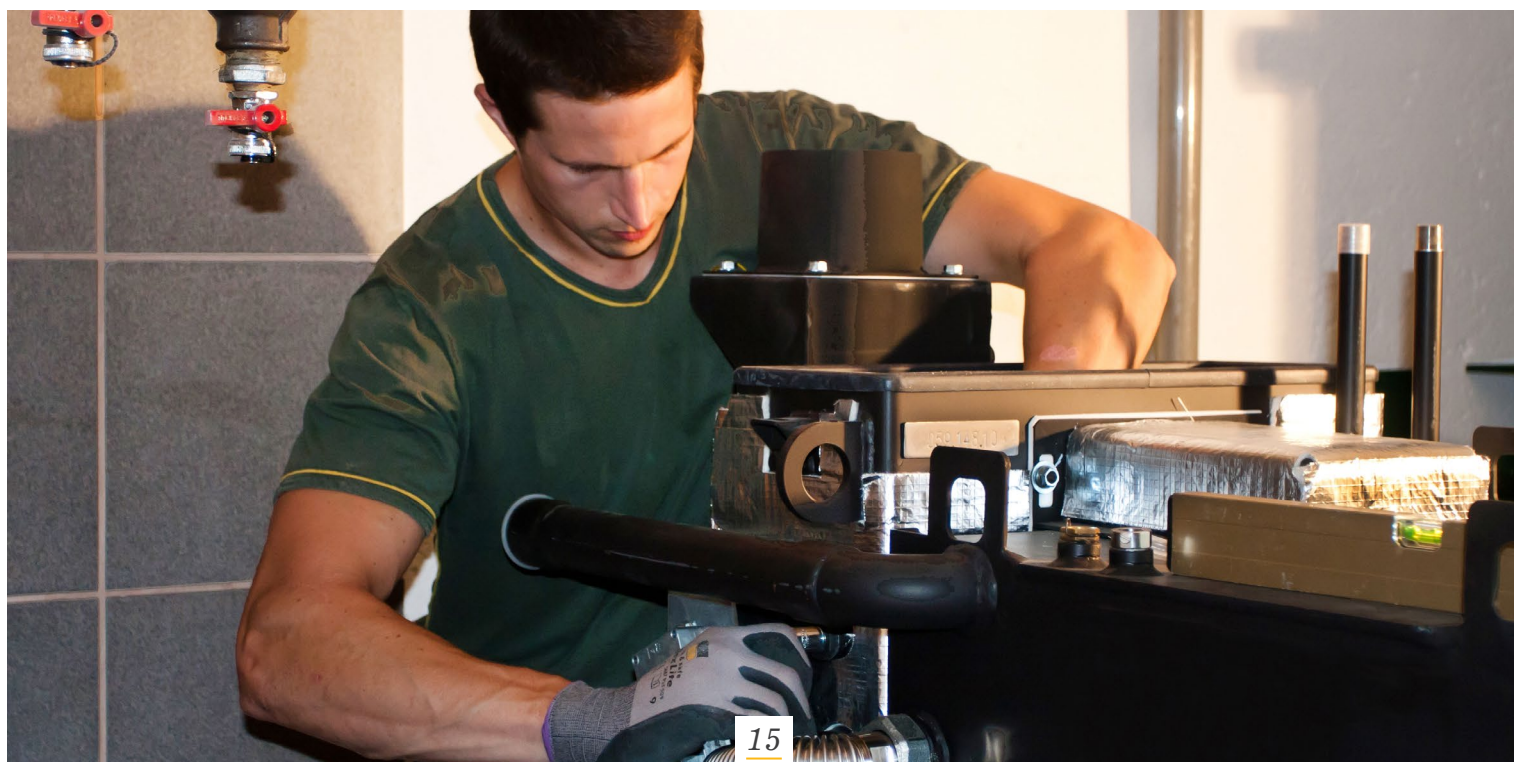
KWB Multifire – Kedel, delbar i 4 dele
